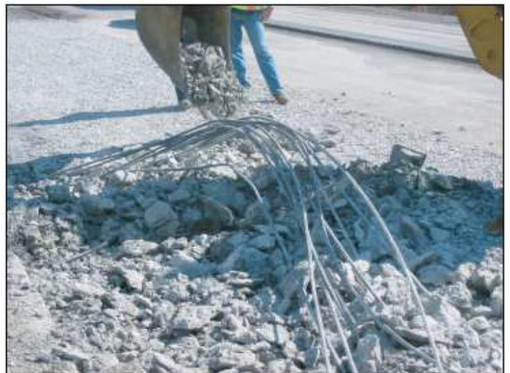
Continuously reinforced concrete pavement
