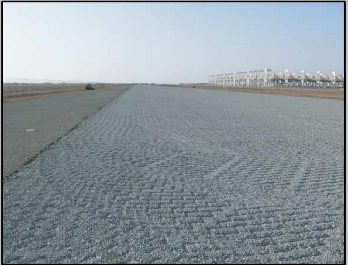
**Existing deteriorated concrete pavement can be effectively modified to create an in-situ structural layer ready to accept an asphalt or rigid overlay.**
