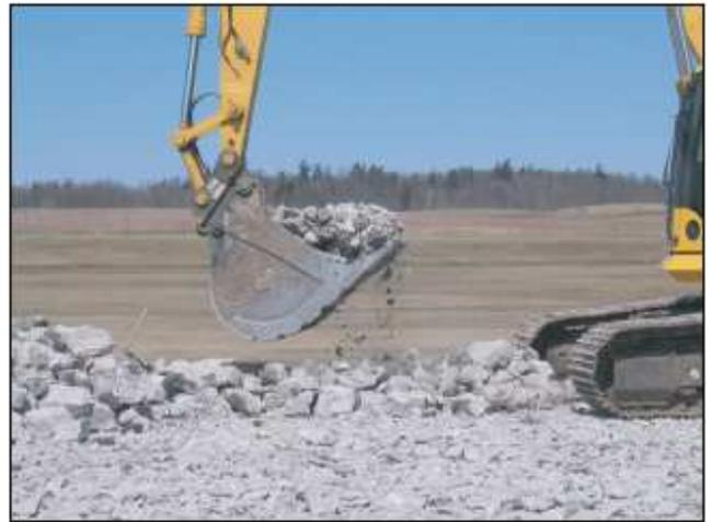
Excavator removing broken jointed reinforced concrete
